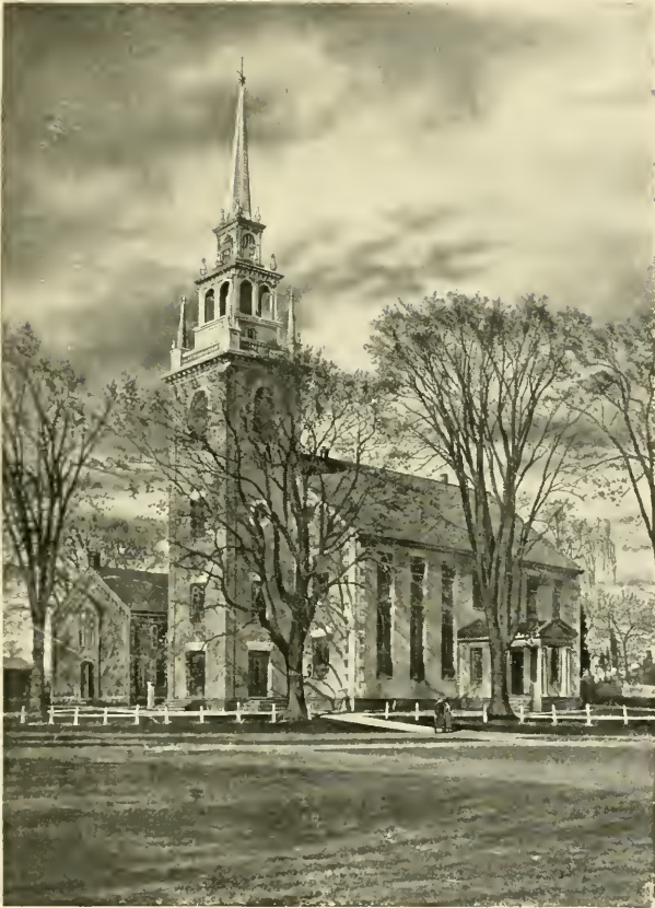
CONGREGATIONAL CHURCH, WETHERSFIELD, CONN. 1761
